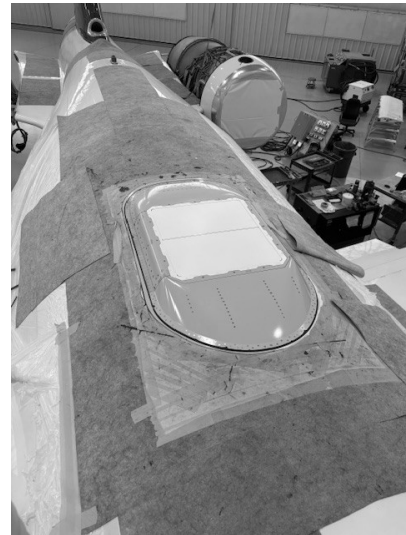
Figure 1. Starlink Antenna During Installation
